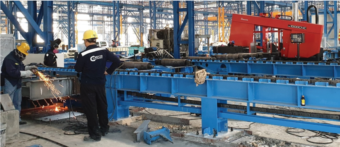
Steel conveyor installation
