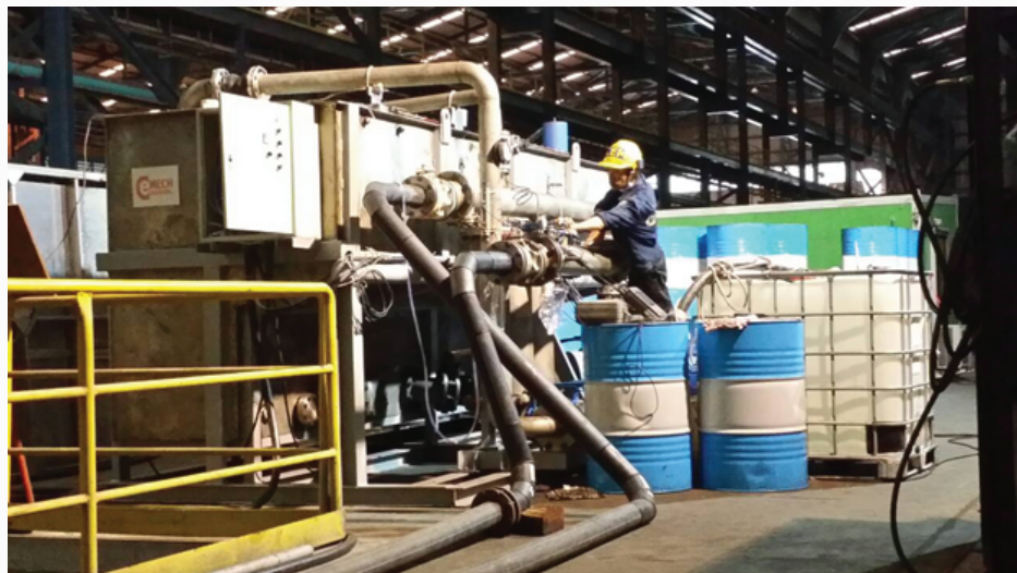
Hot oil flushing work
