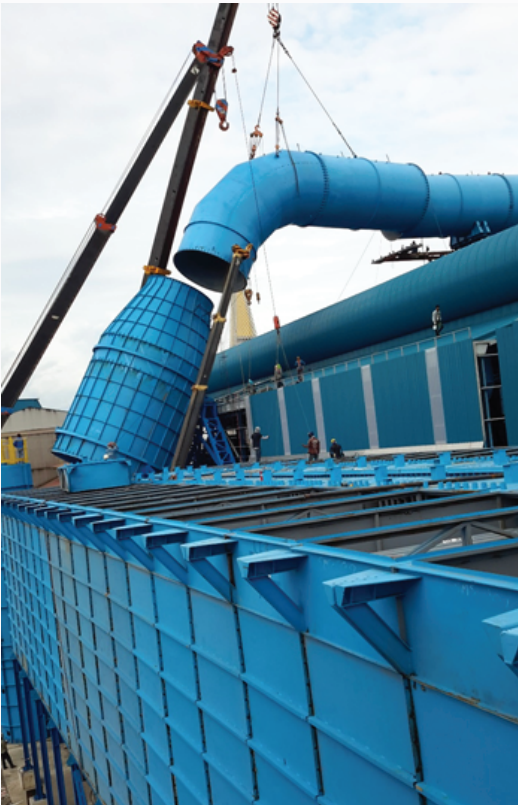
Duct installation
