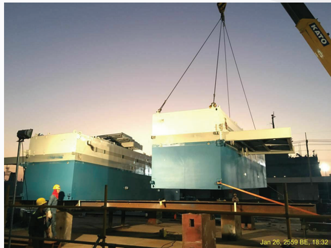
Marin turbine catamaran
