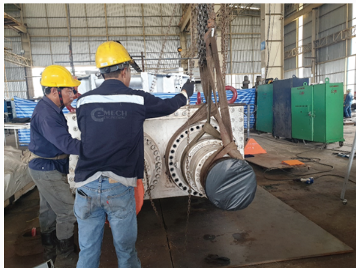
Scrap shredder repairation
