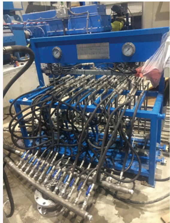
Hot oil flushing work
